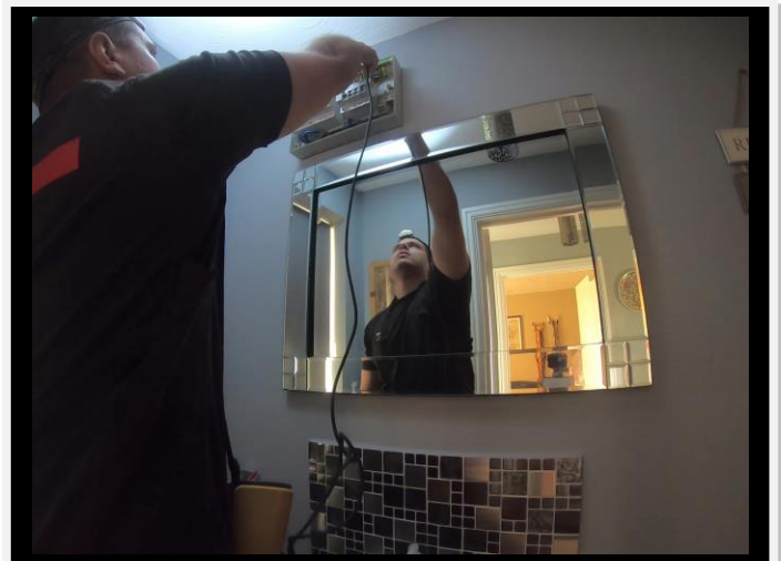
Dom about to carry out Continuity R2 testing to confirm adequate Earth Bonding while carry out an EICR
